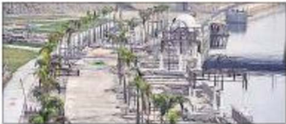
■ Work in progress along the banks of Gomti river in Lucknow.
